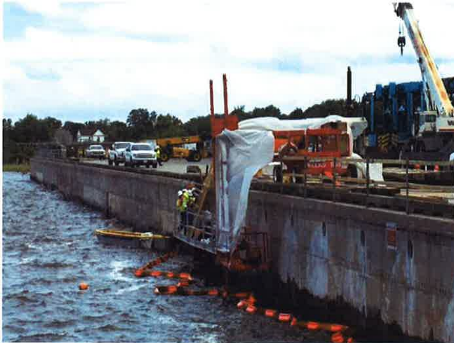
Preparing for the installation of soil anchors
