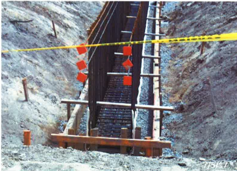
Left: Trench Drain installation between the New North Access Road and Stack 29
