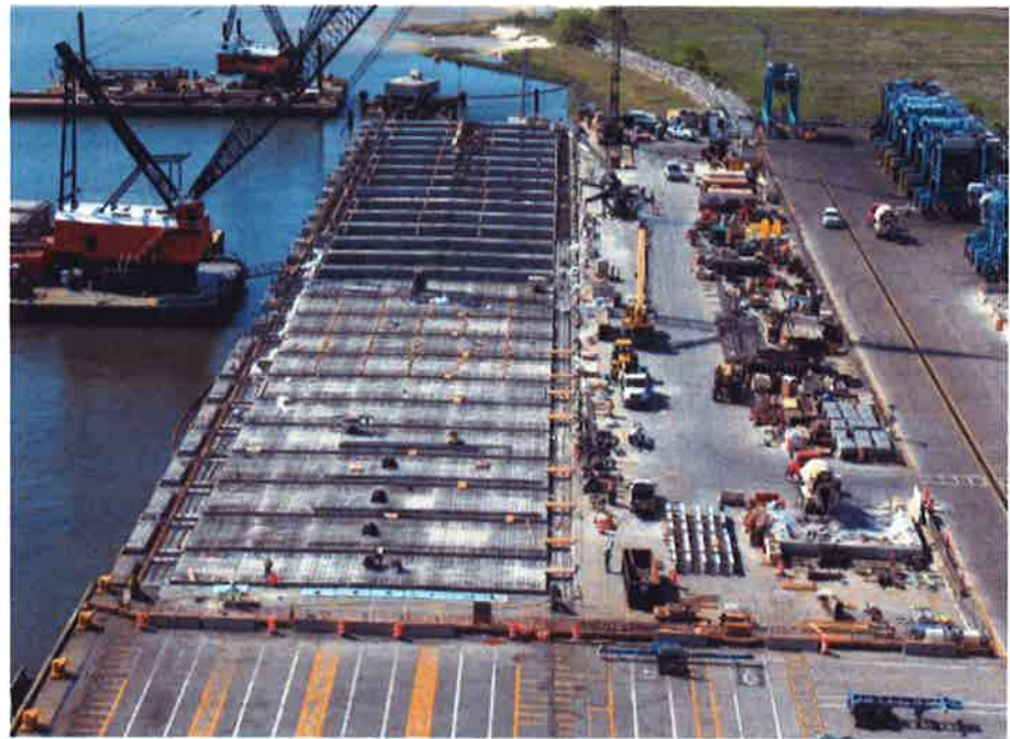
RIGHT: DECKING PLATFORM PLACEMENT
