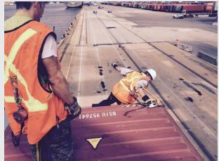
2. Retrieve Rescue Pole with rope and pre-attached hardware from Orange container on Crane.
