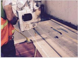
4. Kneel or lay, extend Rescue Pole, Connect Carabiner into D-Ring located on the back of victim's harness and pull the Rescue Pole free. Double check to insure carabiner is securely attached to the victim D-Ring.
